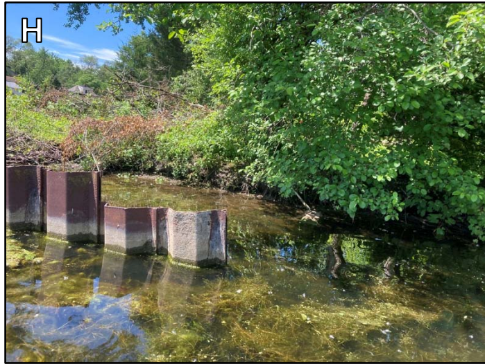
Photo 18. Erosion behind seawall.
