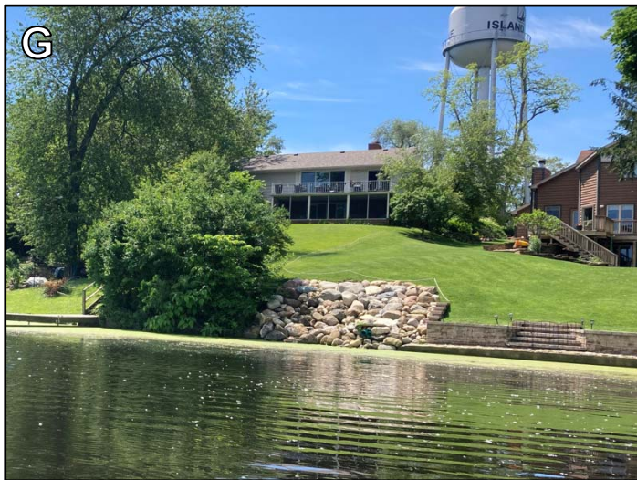
Photo 17. Shoreline repair with rock.
